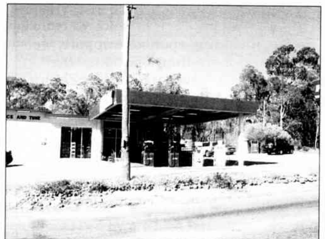
2007 The Peak service station occupies the site today
