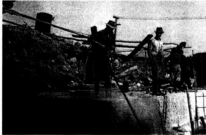
Mr. Albert Grygorcewacz Working On New Wall, 1950
