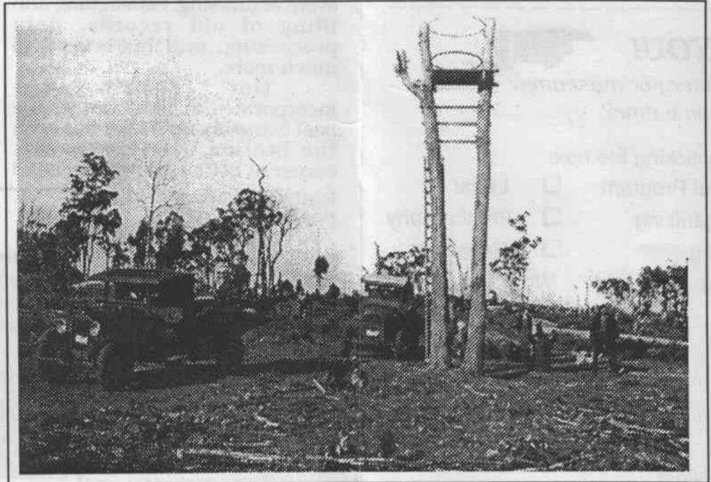
PADDO UNDERDOWN BUILDING THE FIRE WATCH TOWER, SAWYERS VALLEY, CIRCA 1930
